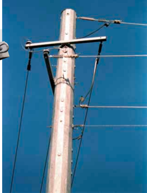
8' braceless 10,000# Dead End assembly, 373' of 795 AAC
