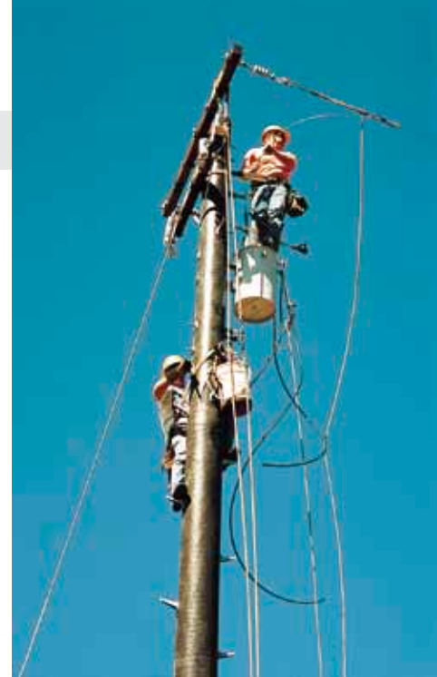
Lewtex® Crossarms being installed on a Shakespeare Composite Structures Tuff-Pole®
